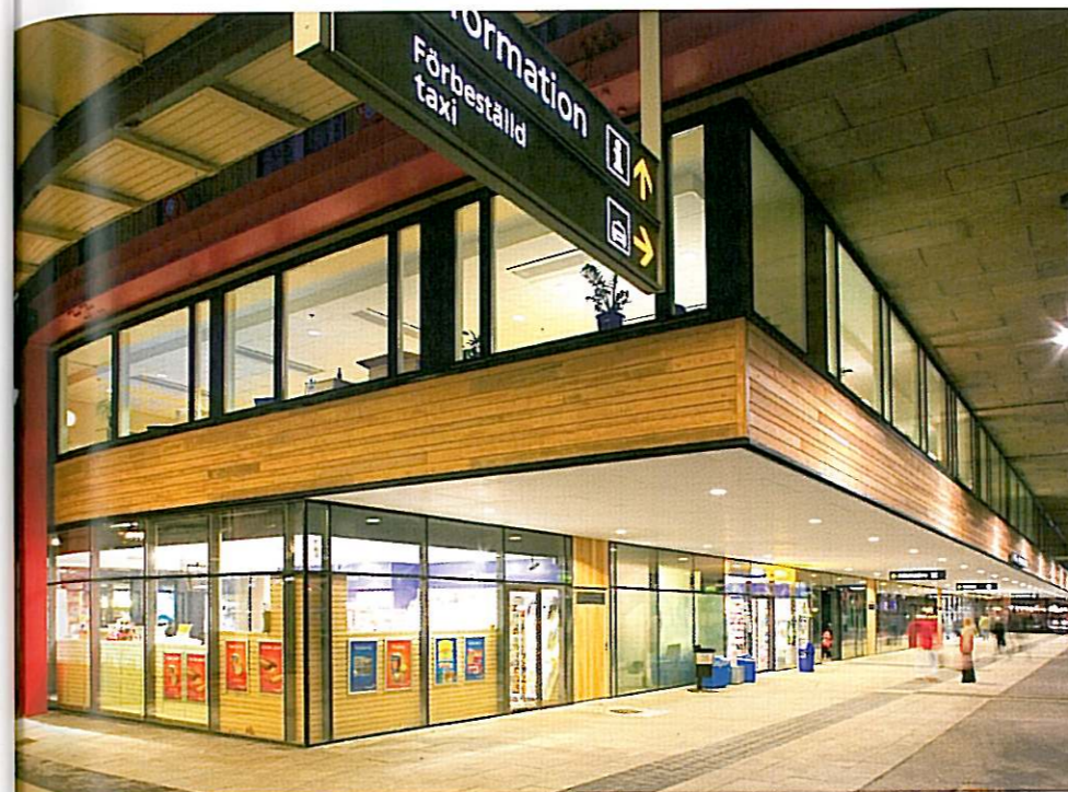
Reisesenteret sett fra plattformssiden. Travel centre seen from the platform side.
